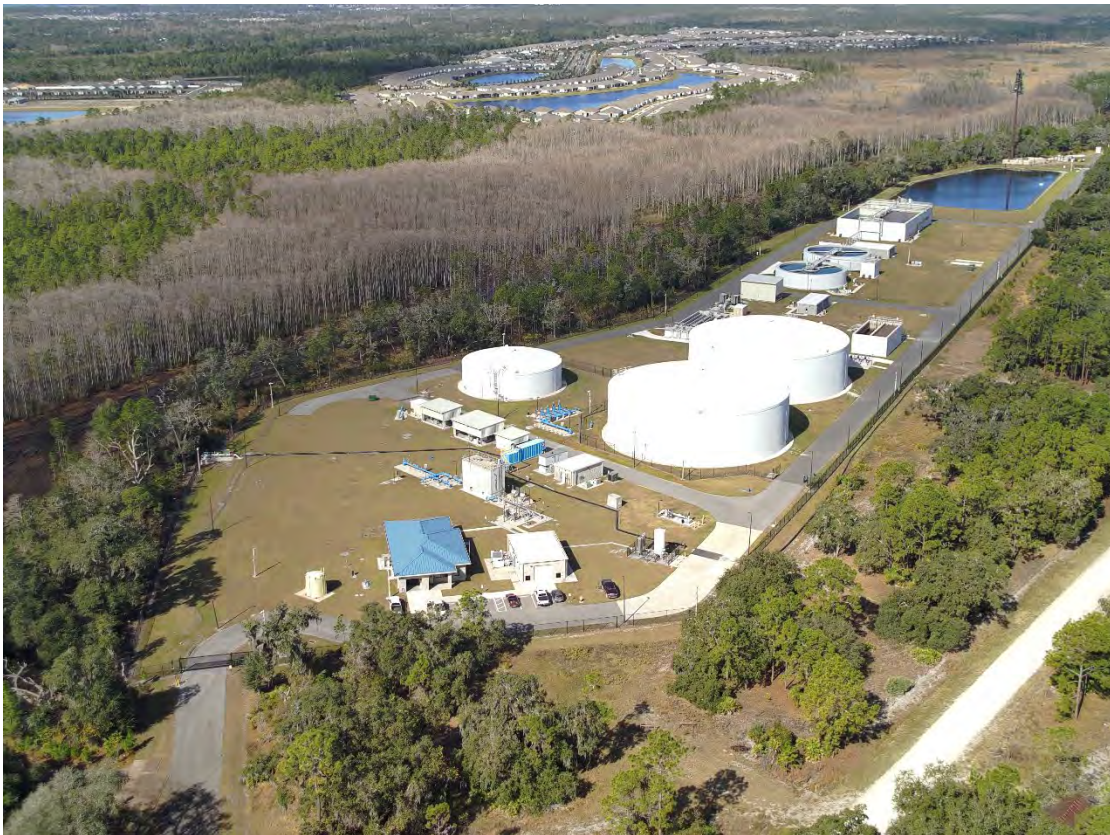
Sunbridge Wastewater Reclamation Facility
