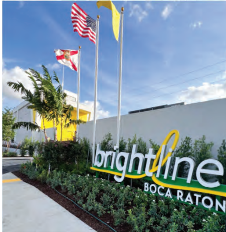
Figure 1 Brightline Station Boca Raton, photo courtesy of the City of Boca Raton
